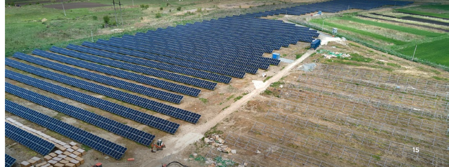
45 MW La Banditella Solar Power Plant in construction, Italy, 2025
